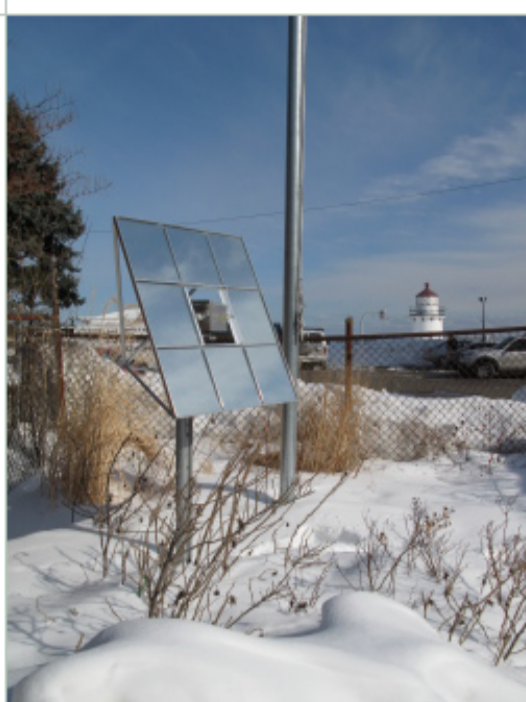
This Practical Solar heliostat at the Tannery Mall in Newburyport, Massachusetts helps brighten several commercial spaces on the north side of the mall.
